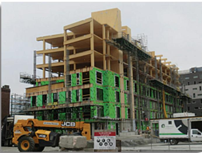
Additional active and passive fire protection features are required to justify the increased height and area for mass timber buildings (Types IV-A, IV-B & IV-C). The proposed changes to this section require this additional protection when these combustible buildings are under construction and, therefore, most vulnerable.
