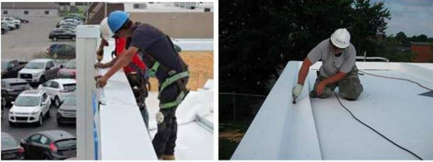
Examples of coped parapets as required by 1503.3.1.
