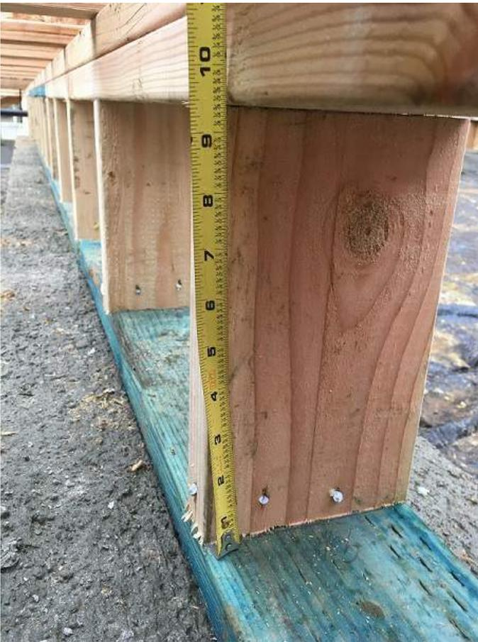
**Cost Impact:** The code change proposal will decrease the cost of construction. This code proposal eliminates the requirement to apply sheathing (e.g. OSB, Plywood, etc.) to interior foundation cripple walls which commonly occur in shallow crawlspaces. Therefore, there is a savings on the material and labor costs to install the sheathing that is currently required in these code sections.
