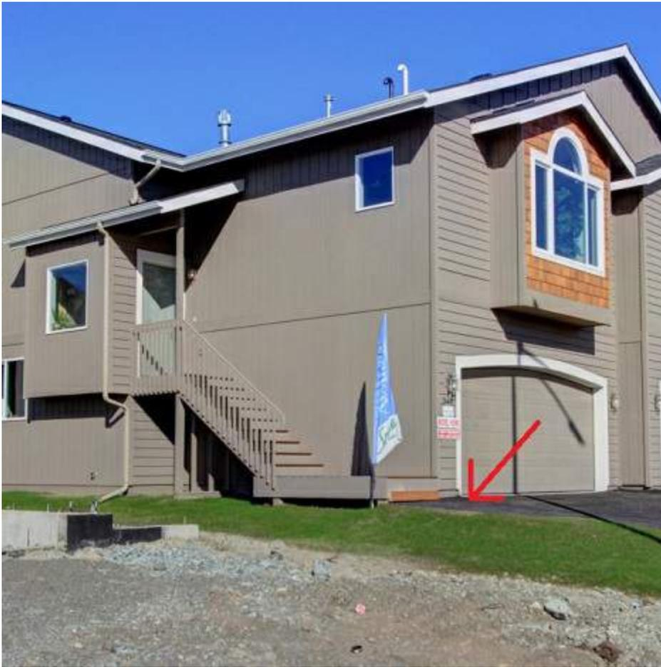
**R401.3 Drainage.** Surface drainage shall be diverted to a storm sewer conveyance or other *approved* point of collection that does not create a hazard. *Lots* shall be graded to drain surface water away from foundation walls. The *grade* shall fall not fewer than 6 inches (152 mm) within the first 10 feet (3048 mm).
