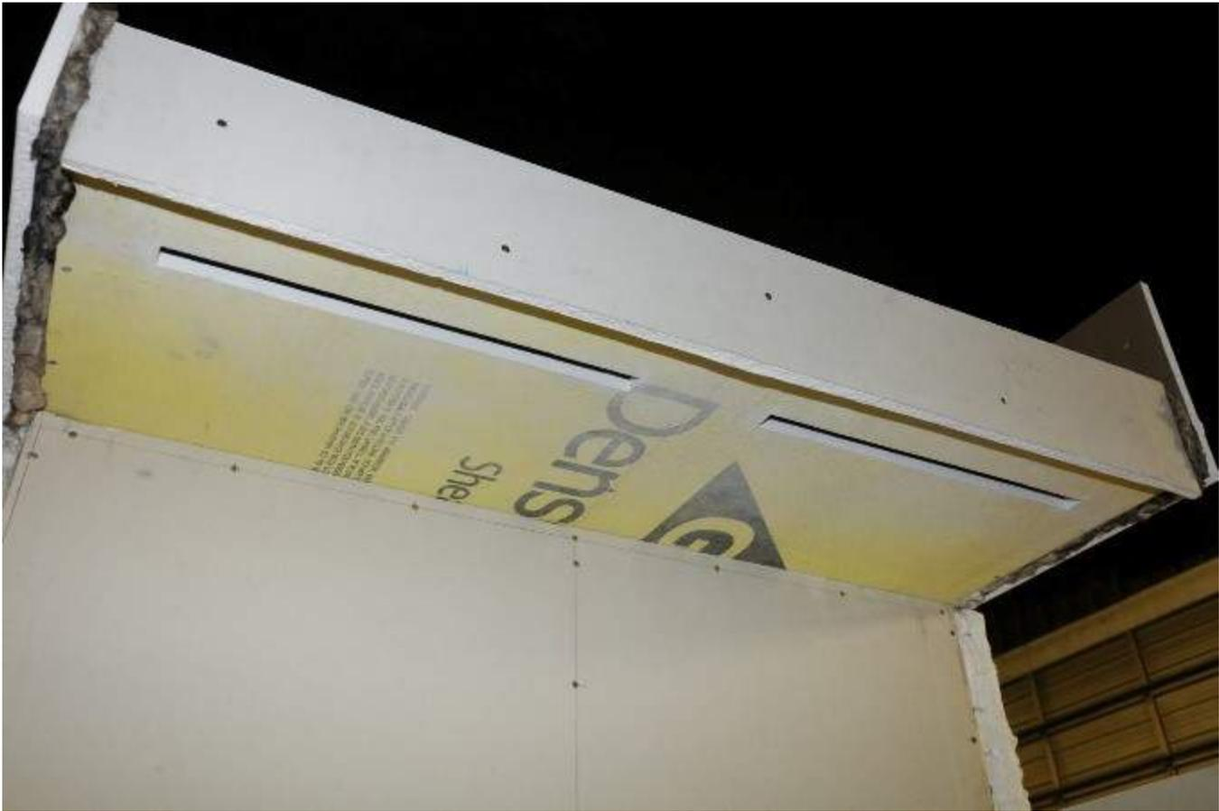
As proposed a 1 hour rated assembly can be used and ventilation would be found in other areas of the roof assembly or a prescriptive vented protected soffit could be constructed. Below is a abstract sketch of a profile of this assembly.
