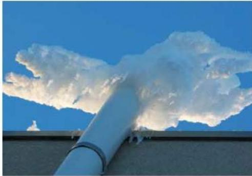
A sidewall termination can also be beneficial in cold climates where water vapor can freeze at the termination of tall, uninsulated systems, closing off the vent.
