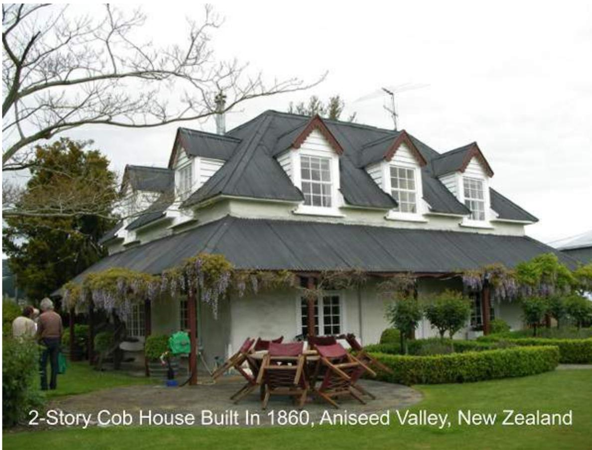
Today, cob is often mixed mechanically using a tractor or mortar mixer, but the wall construction is still generally manual. Cob buildings typically feature raised impermeable foundations and extended roof eaves to protect the walls from moisture and weather. Walls are often plastered with clay, lime or gypsum plasters which protect and beautify the cob without leading to the moisture problems associated with less vapor-permeable finishes such as cement stucco on historic adobe structures.
