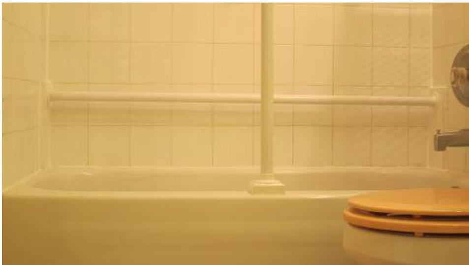
**Figure 2. Bathroom Retrofitted (in a rental apartment)
