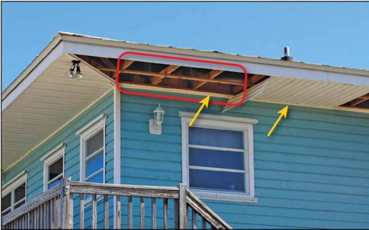
The red outline shows where the soffit panel was stripped from the assembly's J-channel, which remains attached (yellow arrows).
