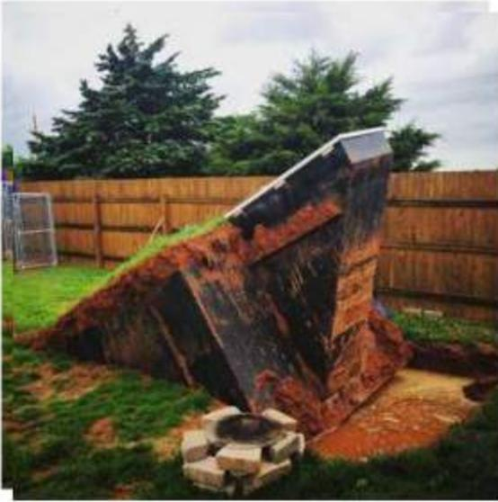
**Figure 2: Failure of an underground residential “storm shelter” not designed per ICC/NSSA-500**
