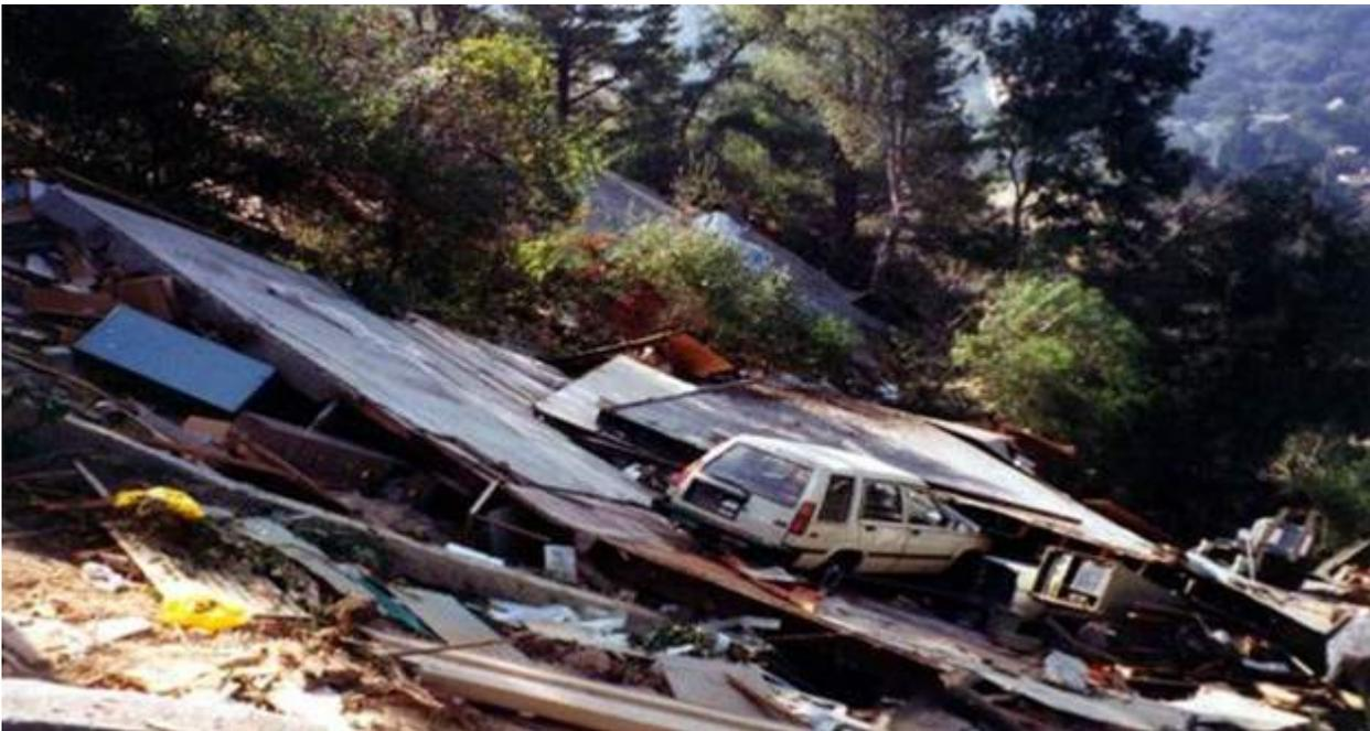
Figure 4. Hillside dwelling collapsed in the 1994 Northridge, California Earthquake (Credit: City of Los Angeles Department of Building and Safety).
