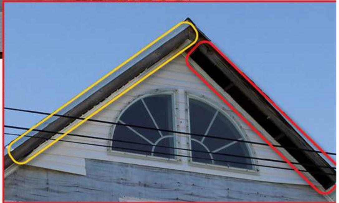
The inset shows the remaining exposed soffit edge on the left side of the ridge (yellow outline) and missing vinyl soffit panels on the right side of the ridge (red outline).
