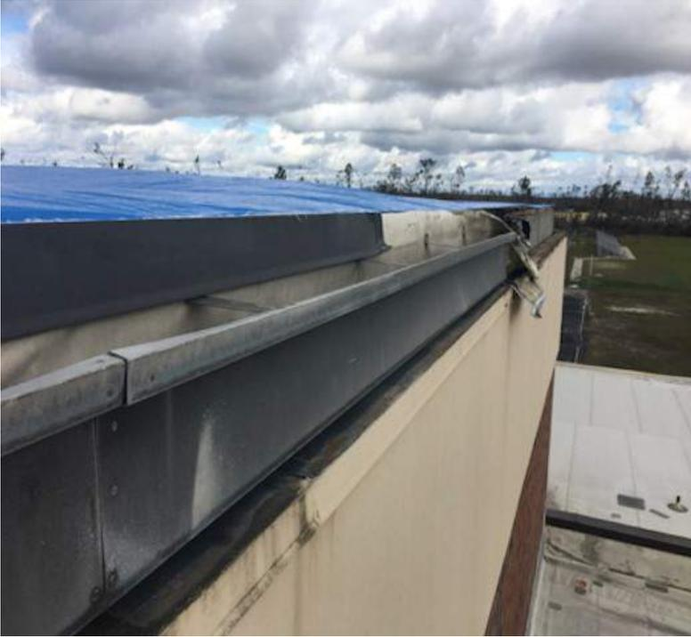
**HICKMAN:** This proposal requires that gutters that are used as part of the edge securement of single-ply roof membranes be tested to the appropriate standard for acceptable wind resistance performance.
