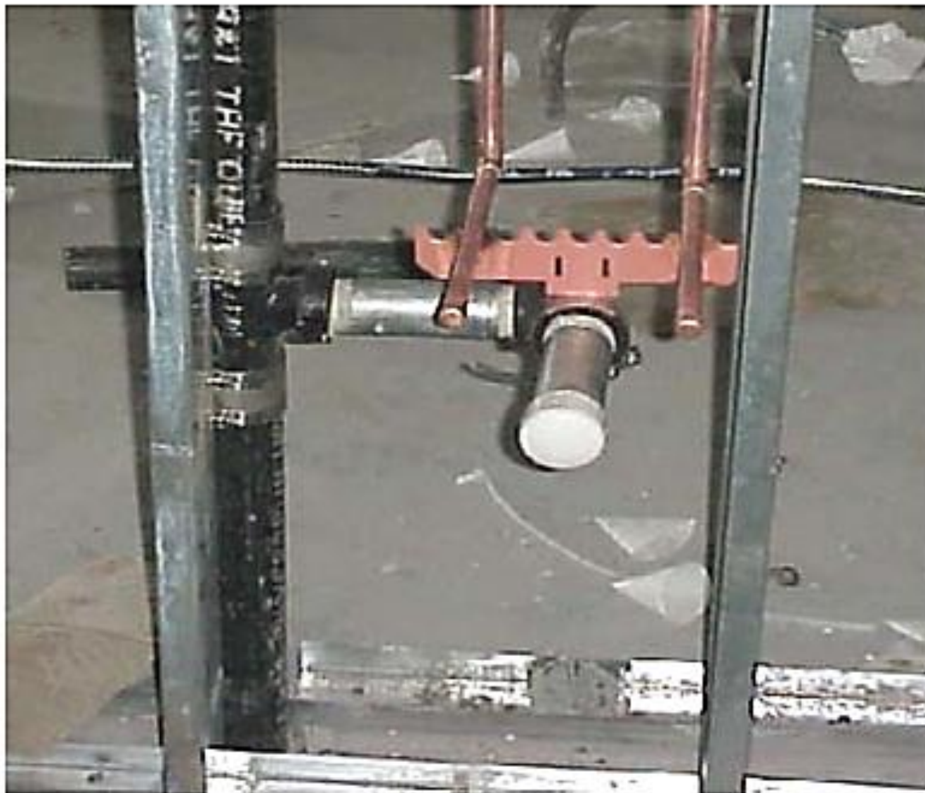
FIGURE 1002.3 "DIRTY ARM" - USE ONLY DURHAM-STYLE FITTING
