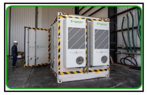
This 1.8MW battery was programmed to be coupled with a previous CHP installation in Puerto Rico and keep the microgrid running smoothly in case of engine failure.
