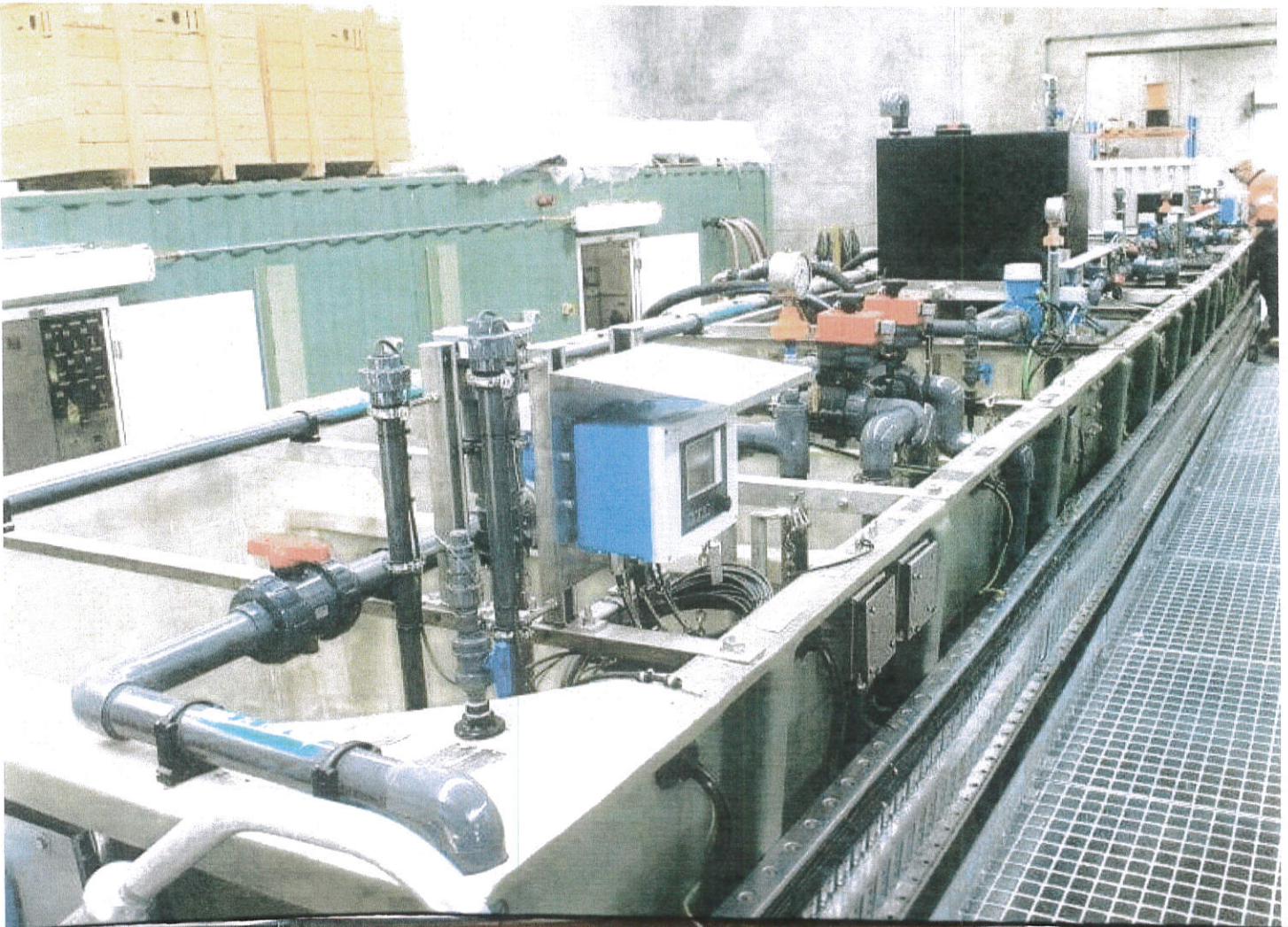
American Falls Plant
