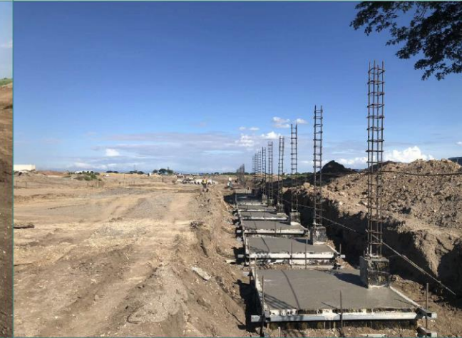
2 Concreting of Footing for Perimeter Fence
