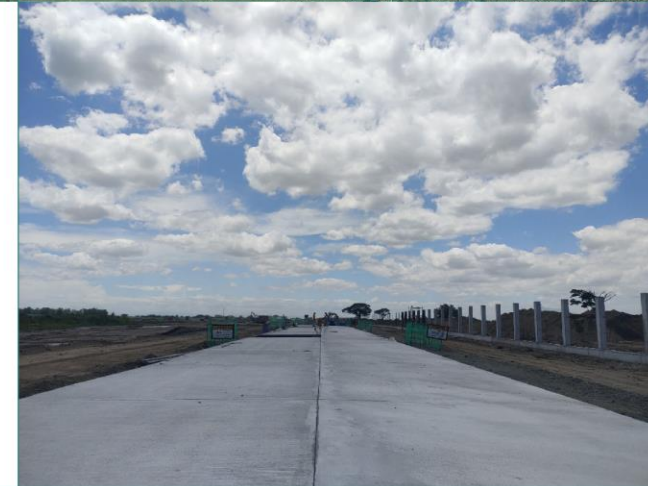
3 PCCP Concrete Pouring 1st Lane
