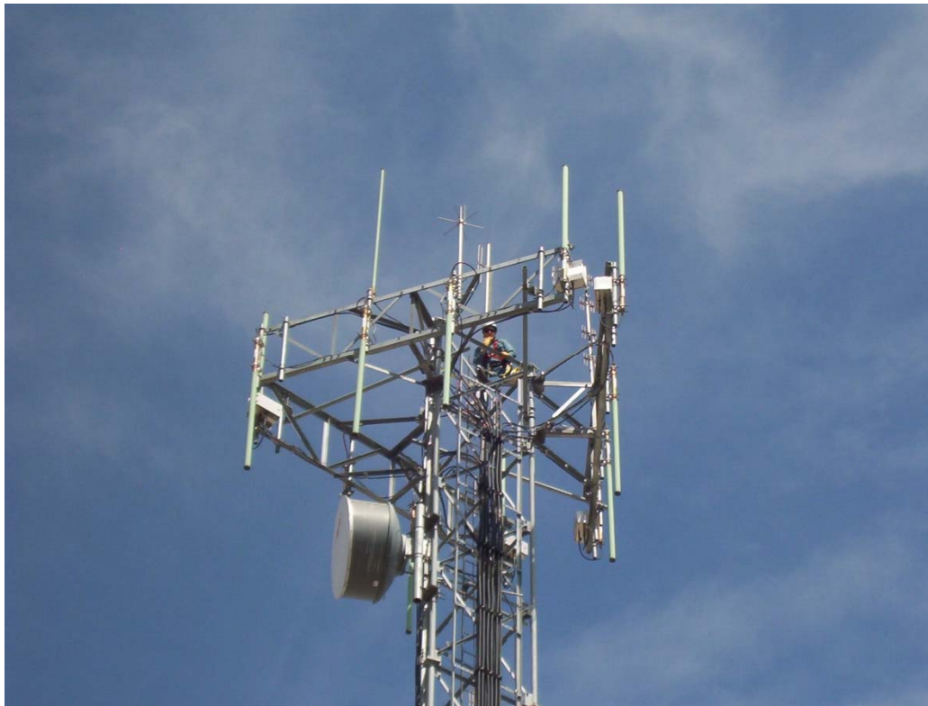
A technician performs maintenance on an RWC communication tower.
