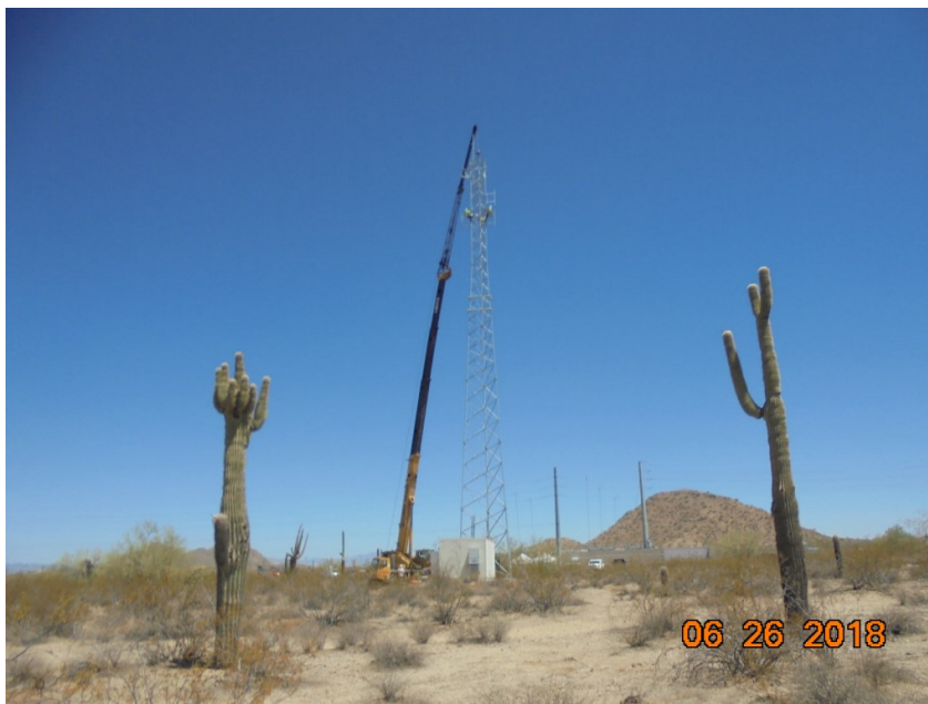
Construction of the new RWC Tower at Pyramid Peak continues.
