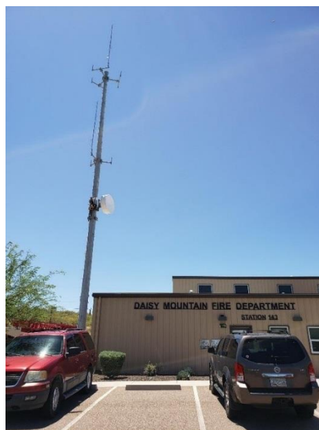
New tower at Daisy Mountain Fire Station 143
