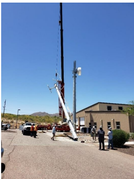
New tower at Daisy Mountain Fire Station 143
