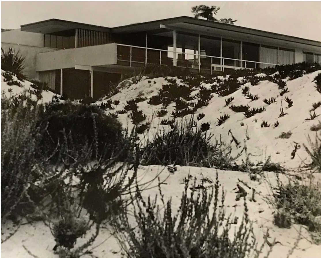
Fig 10. Main View. Arthur Connell, 1957. Reproduced here with the permission of Raymond Richard Neutra, President of the Neutra Institute for Survival Through Design. Original held in the Richard and Dion Neutra Papers, University of California Los Angeles Library, Los Angeles, California. Not for further reproduction.
