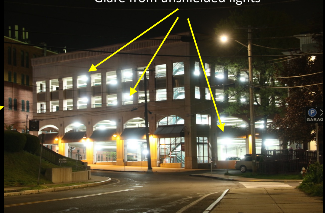
Glare from unshielded lights
