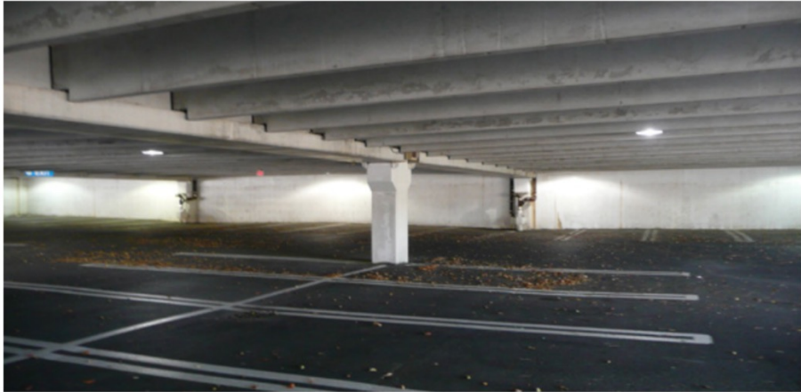
Figure 9(a). Photo of site
