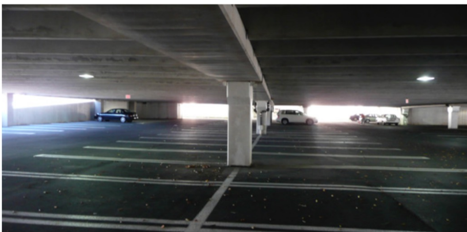
Figure 10(a). Photo of site
