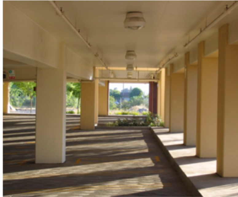
Figure 14. Electric lights off during the day.
