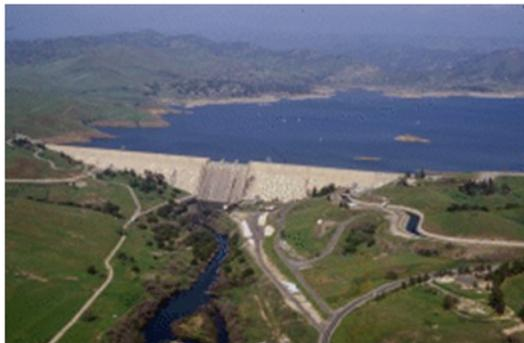
*Friant Dam is a concrete gravity dam on the upper San Joaquin River in the Sierra Nevada foothills of Fresno County, California near the town of Friant. The dam, completed in 1942, forms Millerton Lake and was built by the U.S. Bureau of Reclamation, which owns and operates the dam. BOR photo.*
