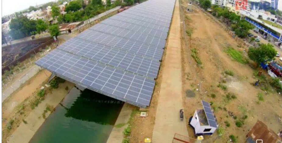
Solar panels covering a water carrying canal in India, yes, that green stuff is water.
