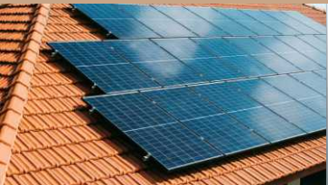
Solar for Common Lighting Solar water Heaters
