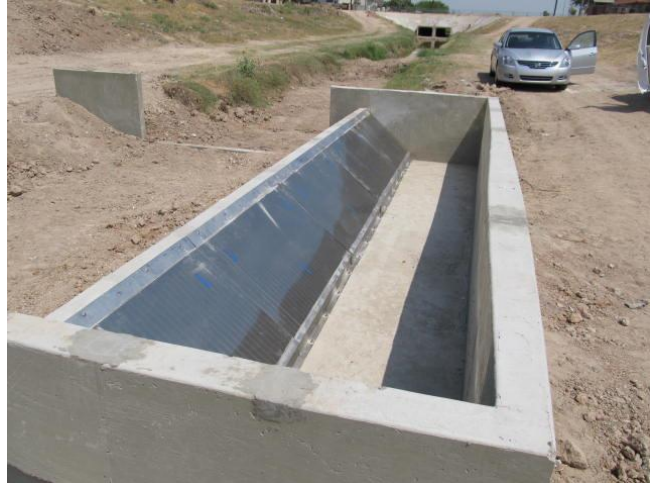
Figure 2. McAuliffe RDF Coanda Screen
