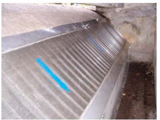
Figure 1 – Curb Inlet Installation
