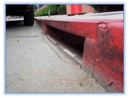
The COANDA Approach Plate, barely visible, fits snug against the curb inlet opening so as not to impede water flow or be exposed to traffic.
