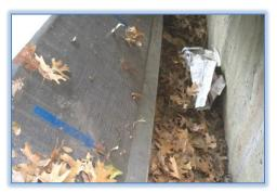
Vector control is not an issue and bacterial growth is significantly impeded because the captured debris remains dry. No special handling techniques are required for debris removal and can be disposed as ordinary municipal waste. Particulate Removal The COANDA filter removes everything larger than fine sand.
