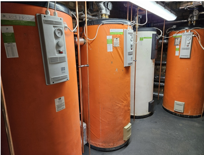
Calorifiers reinstated
