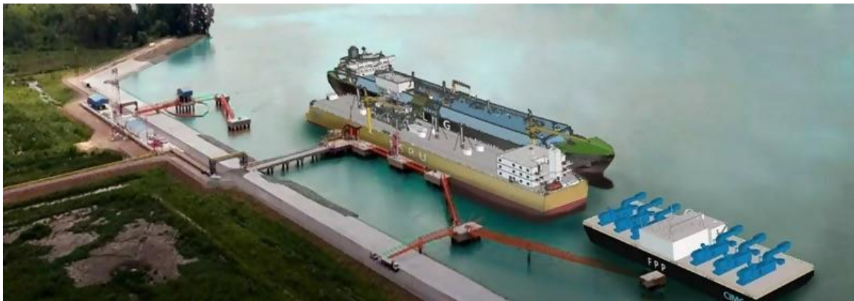
Figure 34 - Power Barge Connected to fuel Supply
