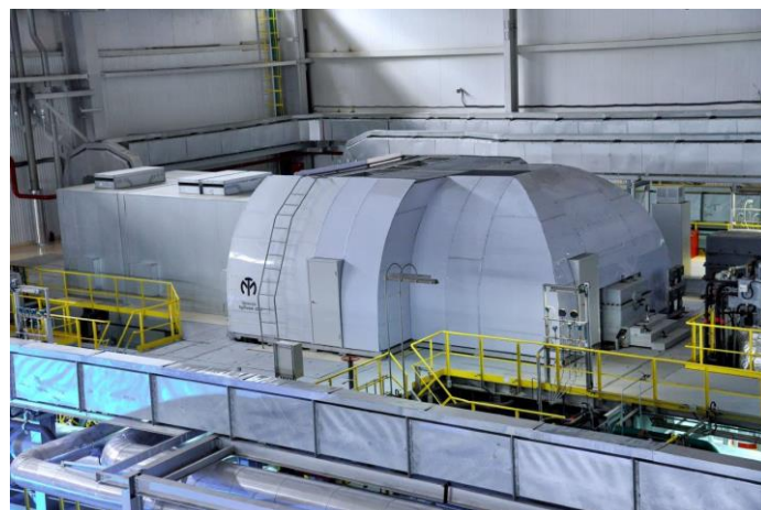
Figure 45 - Gas Turbine Housing
