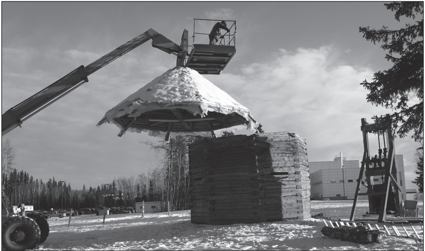
Figure 4: The spruce pole roof from 1982 being removed from the blockhouse in 2010.
