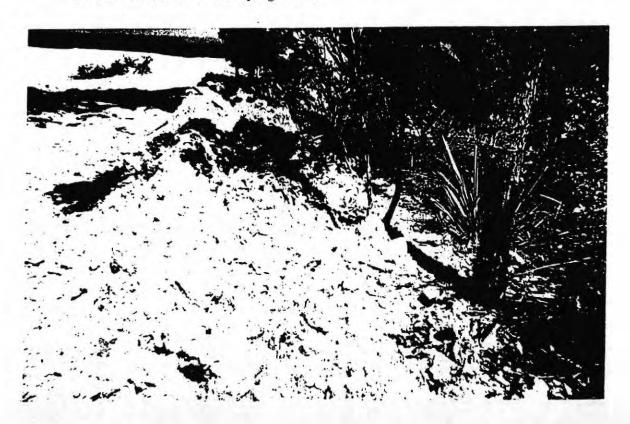
PLATE 2 Dry weather survey. A more substantial portion of the bund along the northern boundary, illustrating extremely limited discharge of sediment into the adjacent bushland. There is no evidence for a reduction in plant vigour adjacent to this bund.
