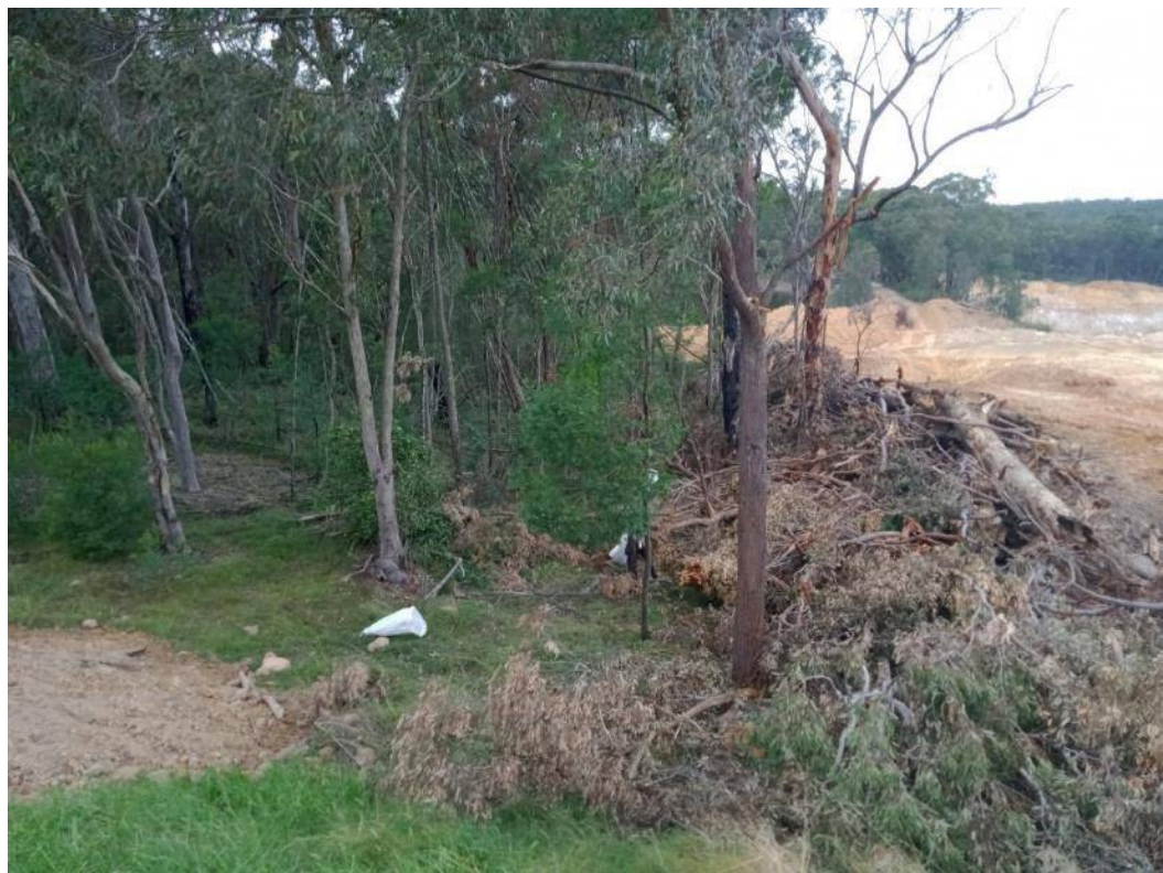
Figure 4: Disturbance to east boundary of Lot 1 after quarry works in May 2020
