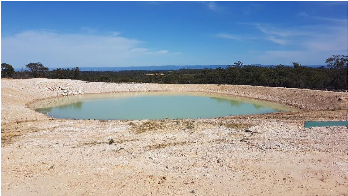
Image 4. Extraction area stage 2 dam construction site
