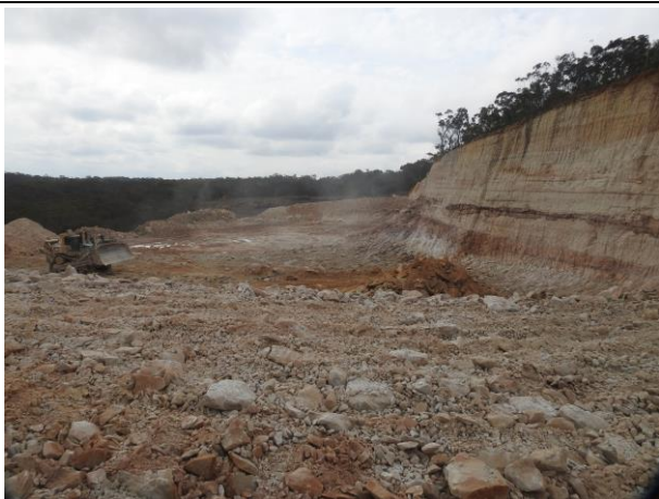
Photo 15: Ripping sandstone in Stage 1B (1022B_0024)
