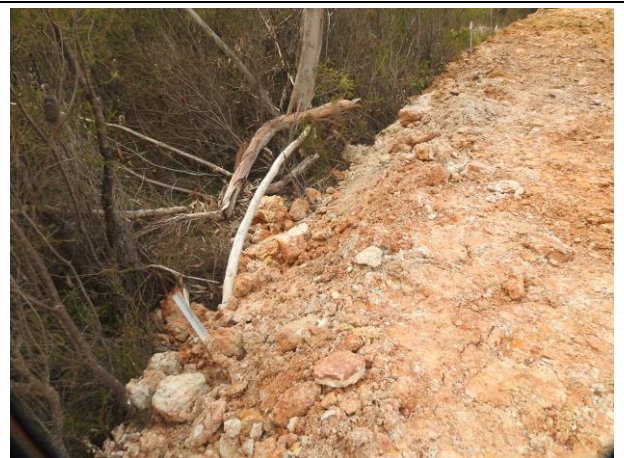
Photo 12: A boundary peg partly buried by the bund wall constructed on the western boundary of Stage 1A (1022B_0016)
