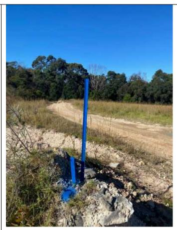
Plate 7: Metal picket installed at survey timber marker, Lot 2 southern boundary.
