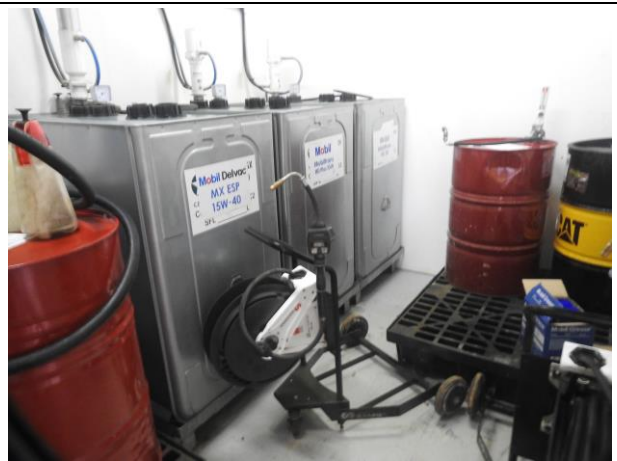
Photo 2: Self-bunded hydrocarbon containers and 205L drums on bunded pallets in active area workshop (1021B_0009)
