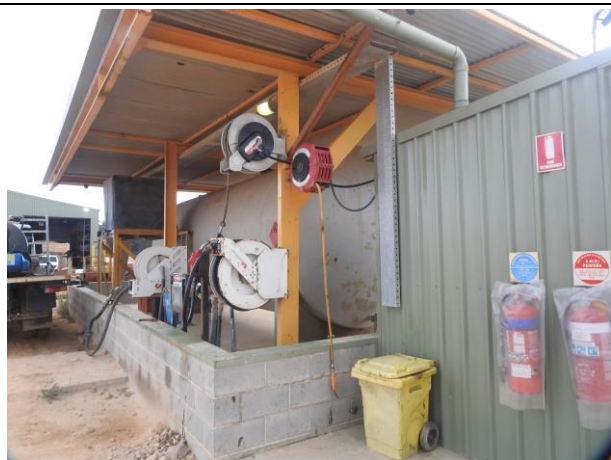
Photo 5: Main bunded diesel storage tank (1021B_0018)
