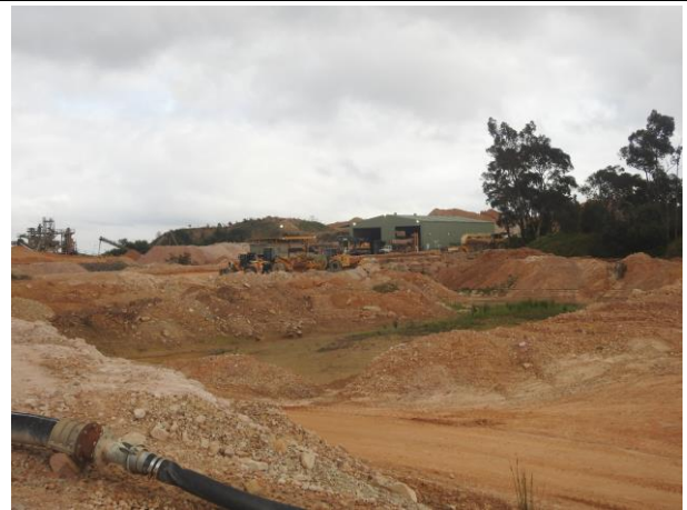
Photo 10: Silt Dam 3 used for mud clean up (1021B_0026)
