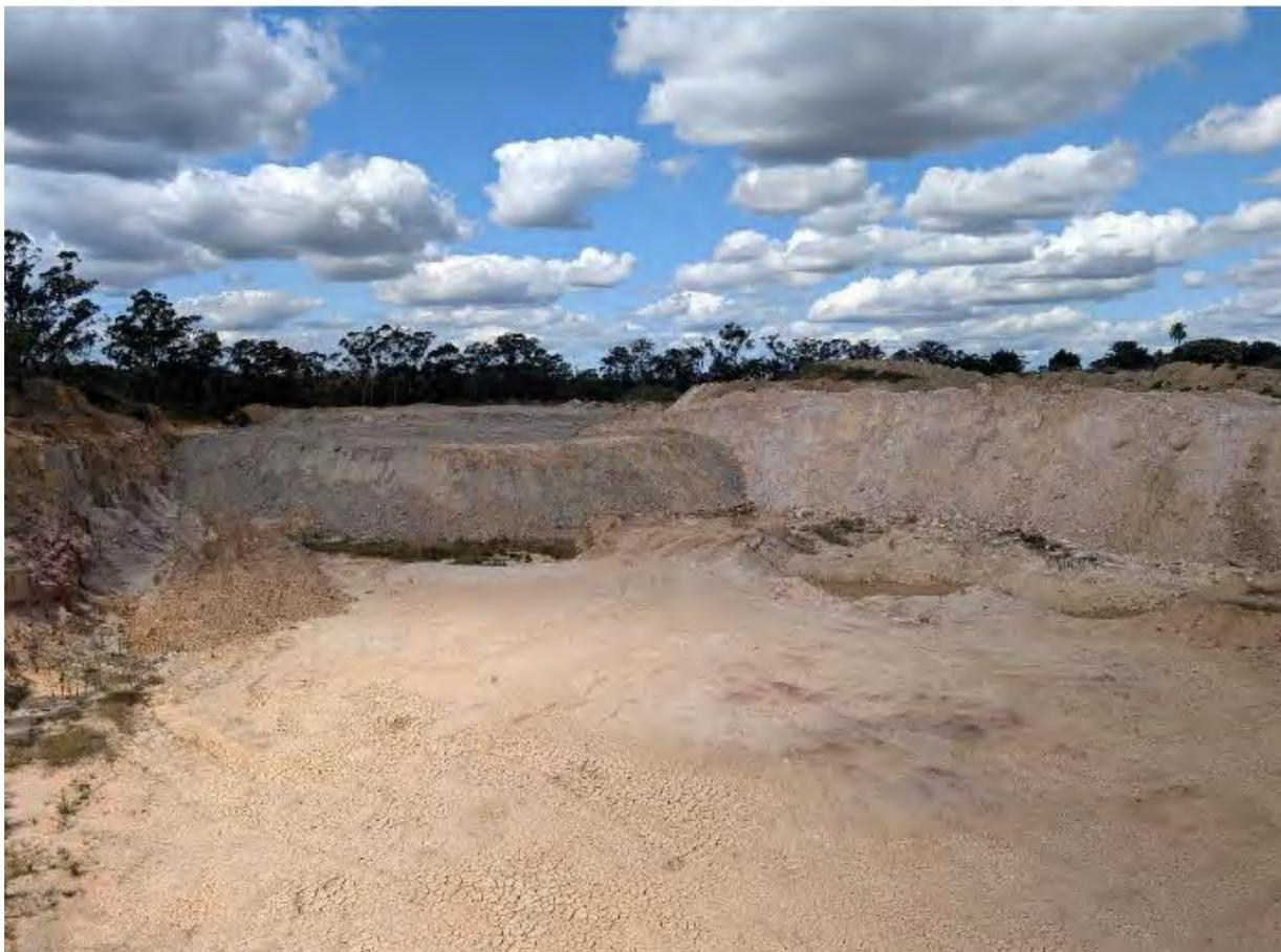
**Plate 1 – Commencement of final landform shaping in Stage 1 Extraction area (South East Environmental 2024).**
