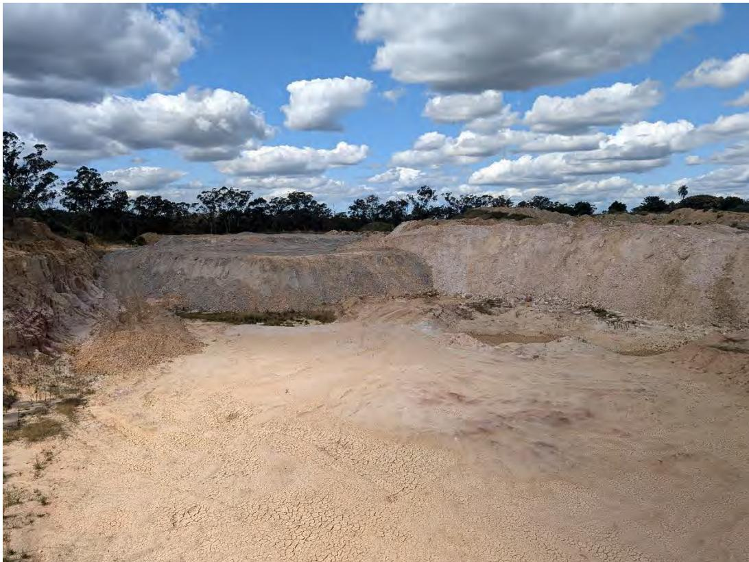
**Image 2.** Extraction area stage 1 with rehabilitation material raising the ground level to final contour height
