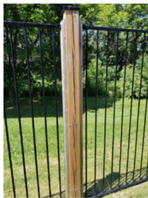
Figure 5. A wrought iron fence without cross rungs is more difficult to climb.
