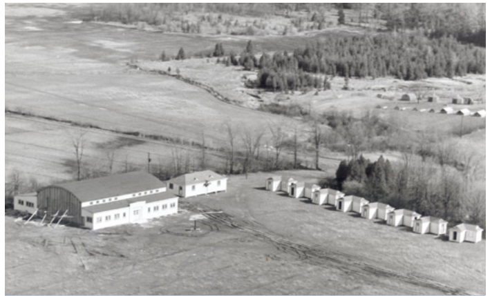
Aerial shot of Bandberg under construction, n.d. K-W Record Photo, Ellis Little Local History Room, Waterloo Public Library, WatPL 31601
