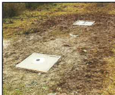
Concrete pad and steel wellhead protection cover for paired wells at ground surface.
