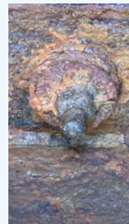
Steep Creek Bridge - Uncoated
