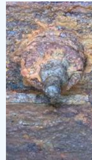
Steep Creek Bridge - Uncoated
