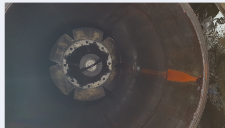
Figure 9 - ILI Run with no debris in receiver
