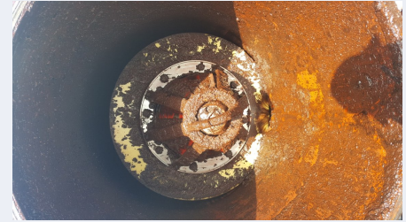
Figure 7 - Heavy Duty Cleaning Pig - T2+ Cleaning Run
