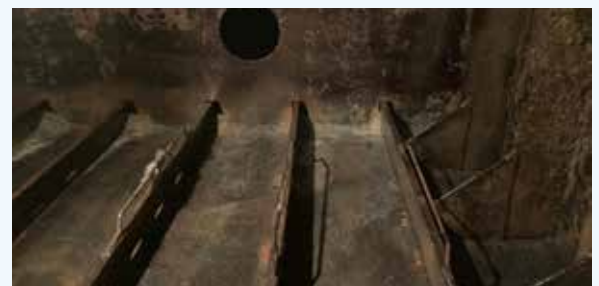
Ballast tank coated in S2S
