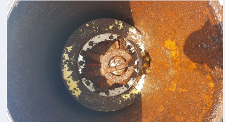
Figure 7 - Heavy Duty Cleaning Pig - T2+ Cleaning Run
