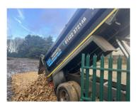
The extensive removal of brambles significantly disturbed the ground, resulting in an extremely boggy and unstable surface. This made the working conditions unsafe for further activity. To address this, 96 tonnes of hardcore had to be laid down to stabilise the area before any work could safely commence. Drainage & Weed membrane was also applied to pathways
