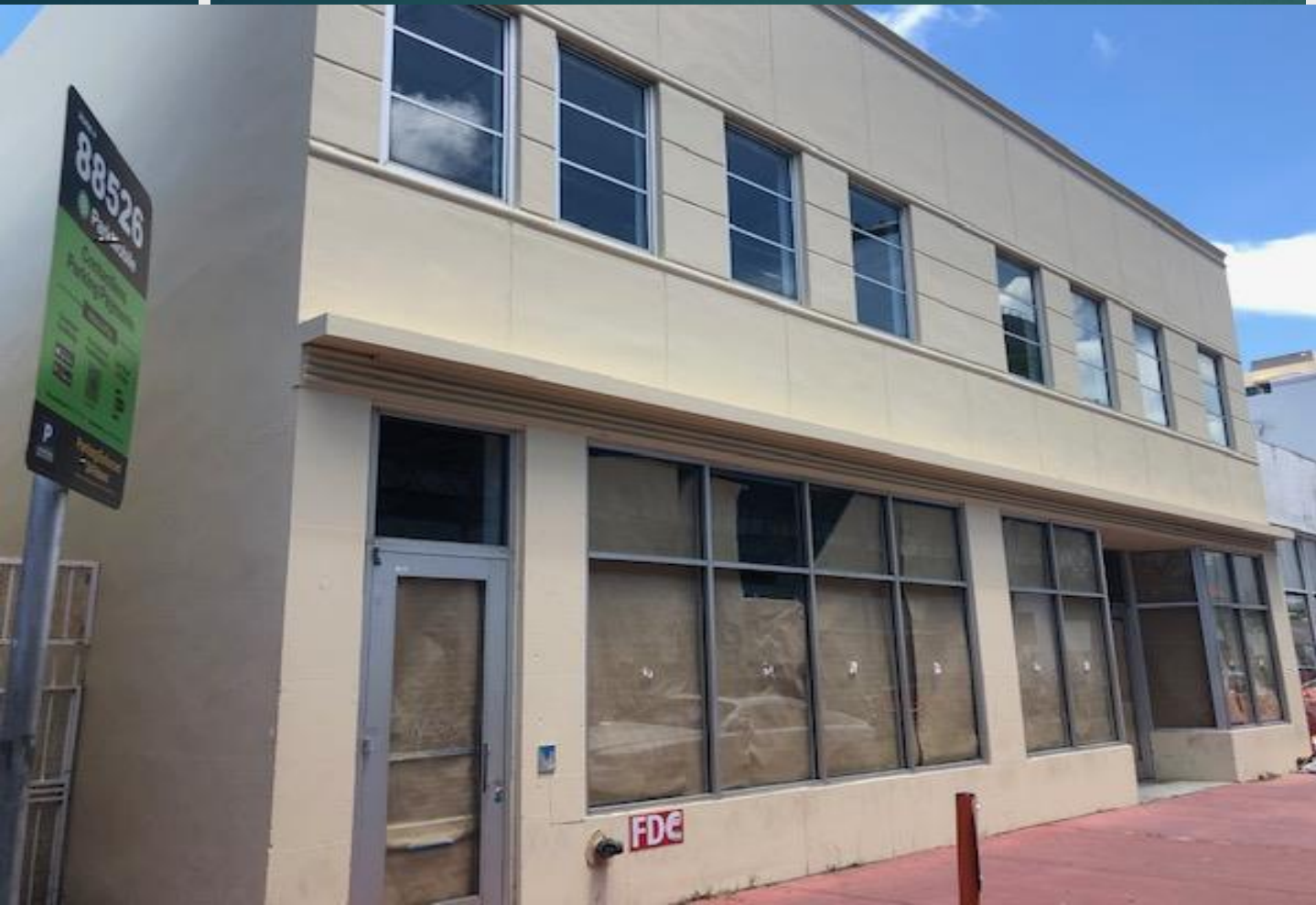
2 Front doors and 1 back door.
