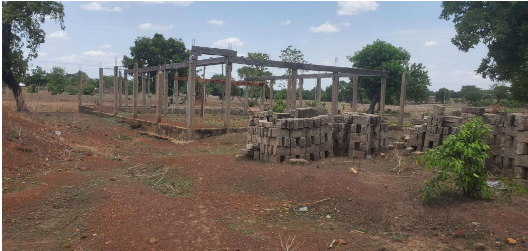
Tindoma church building project started by Elizabeth has come to a standstill due to loss of her job
