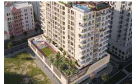
Project : The Hub Residences MEP Consultant : Kaizen Architects & Engineers MEP Contractor : Gamma Contracting LLC Location : Al Furjan, UAE Year : 2025
