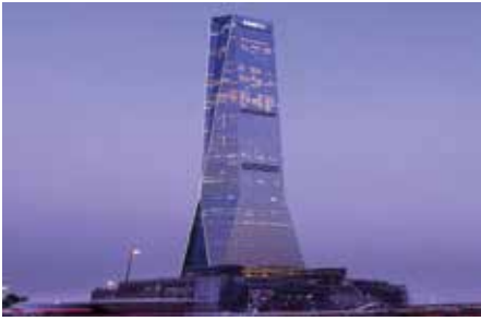
Project : SO/ Uptown Dubai Hotel & Residences MEP Consultant : WSP MEP Contractor : Voltas Limited Location : Dubai, UAE Year : 2023
