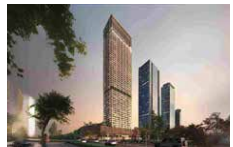
Project : Saba-4 Tower MEP Consultant : LACASA Architects & Engineering Consultants MEP Contractor : Prime Star Electrical And Mechanical Works LLC Location : JLT-Dubai, UAE Year : 2025
