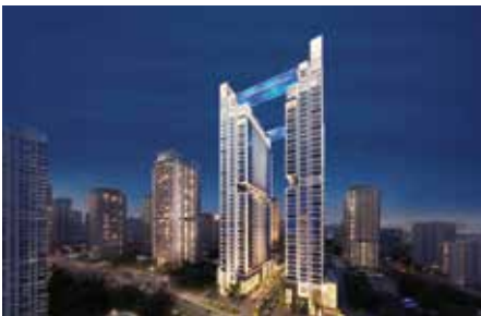
Project : Viewz 2 by Danube Commercial & Residential Building MEP Consultant : National Engineering Bureau MEP Contractor : Al Andalus Power Electromechanical LLC Location : Dubai, UAE Year : 2024
