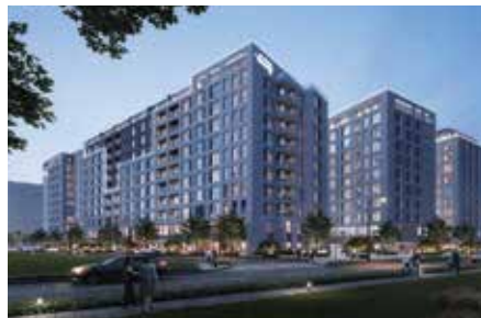
Project : Al Mamshah Seerah Residential Phase 1 MEP Consultant : Mimar Architecture & Engineering MEP Contractor : E7M Electromechanical Works Contracting LLC Location : Sharjah, UAE Year : 2024
