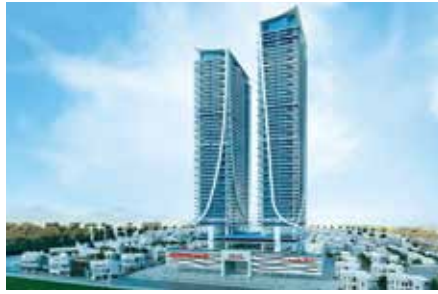
Project : ELITZ 1 Tower by Danube MEP Consultant : Al Khawaja Engineering Consultancy MEP Contractor : EMAC Electromechanical LLC Location : Dubai, UAE Year : 2024
