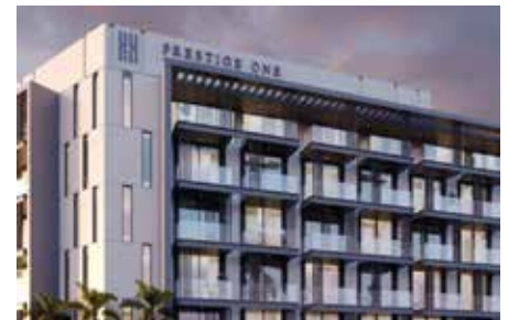
Project : The Residence by Prestige One MEP Consultant : Model Engineering Consultants MEP Contractor : ANJ Expert Electromechanical LLC Location : Dubai, UAE Year : 2025
