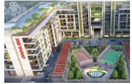
Project : Petalz by Danube MEP Consultant : National Engineering Bureau: NEB MEP Contractor : Al Andalus Power Electromechanical Works LLC Location : Dubai, UAE Year : 2024
