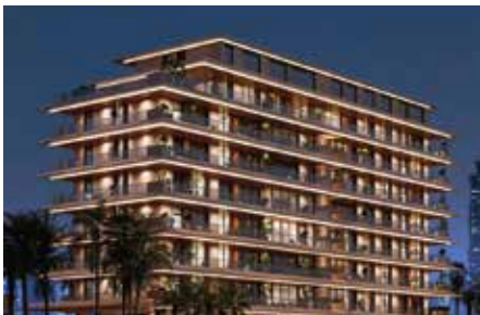
Project : Canal Residential Project MEP Consultant : Dewan Architects & Engineers MEP Contractor : IZone Electromechanical Contractors L.L.C Location : Al Wasl, Dubai, UAE Year : 2025
