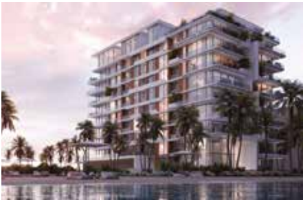
Project : Luce (2B+G+9+R) Residential Building MEP Consultant : MZ Architects MEP Contractor : Al Ashram Contracting LLC Location : Dubai, UAE Year : 2024
