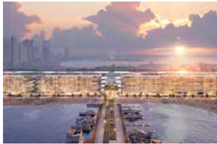
Project : Dubai Harbour Residences by Shama Holding MEP Consultant : SSH Design MEP Contractor : Khansaheb MEP Location : Dubai Harbour Zone 4, Dubai, UAE Year : 2025
