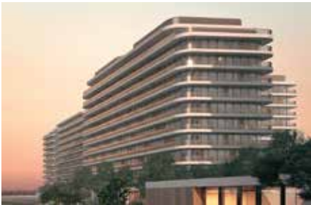
Project : Eden House – The Park MEP Consultant : Erga Progress Engineering Consultants MEP Contractor : Bilt Middle East (MEP Division of Al Basti & Muktha Group) Location : Al Wasl, Dubai, UAE Year : 2025
