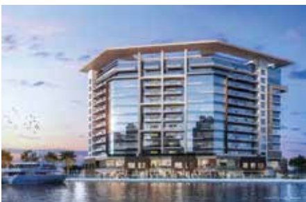
Project : Residential Building At Plot C33 Yas Island MEP Consultant : Khatib & Alami and Partners Consulting Architects & Engineers MEP Contractor : Anson Construction L.L.C Location : Abu Dhabi, UAE Year : 2025
