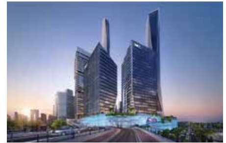
Project : DMCC Uptown Phase 2 T3 & T4 MEP Consultant : Samadhin+ Associates Consulting Engineers MEP Contractor : Menasco Mechanical Contracting Co LLC Location : First Al Khail Street, Dubai, UAE Year : 2025
