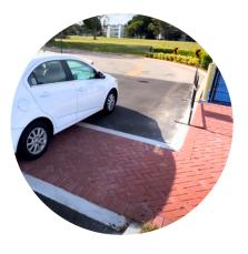
Near the parking lot pickleball complex, we have installed a new speed table and paver crosswalk to offer a safer passage for pedestrians to and from these facilities. In addition to the added safety of this roadwork, it makes the area more appealing, connecting the parking lot courts to the rest of the clubhouse amenities.
