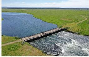
Grand Centennial. The new bridge arrived at Harriman State Park in three sections on October 28, 2020. It was assembled on shore over the next two days while the crane operators spent the following weekend moving three cranes on site for the lift and set. On November 2, 2020, the new Ranch Bridge was laid in its final resting place. On June 15, 2021, FHSP and Harriman State Park hosted a dedication and Centennial Celebration rejoicing in this achievement.
