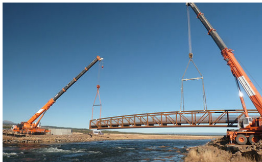
New bridge placement. Photo courtesy FHSP
