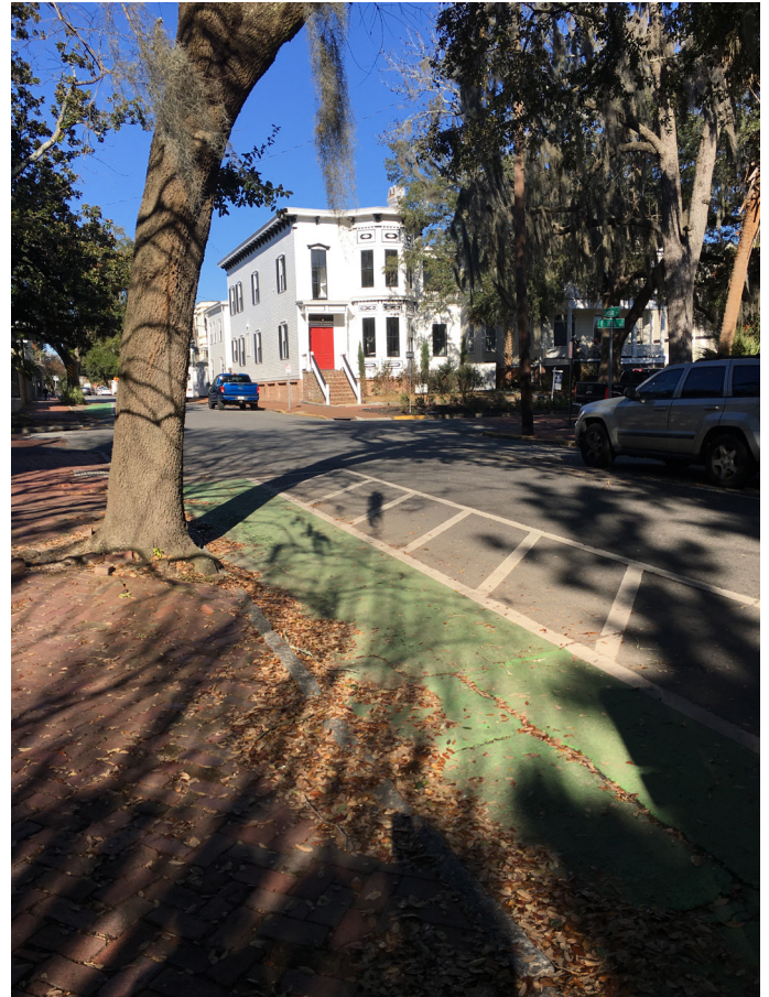
Intersection of East Hall and Lincoln Street
