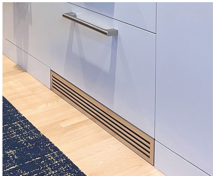
REFRIGERATOR VENTED TOE KICK
