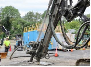
the Northeast. Geo-CoE will create mobile platforms consisting of thermal exchange manufacturing equipment and trained personnel—like those pictured above—that can be deployed to build thermal exchangers where needed. [Photos courtesy of Eversource.]
