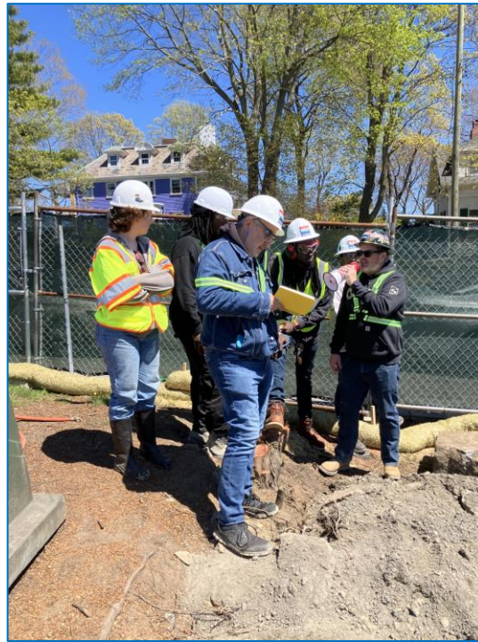
Students in GDA's Spring 2025 Geothermal Drilling Intensive learn from expert trainer Brock Yordy about the equipment, crew, and activity they are witnessing on the active drill site of Skillings & Sons.
