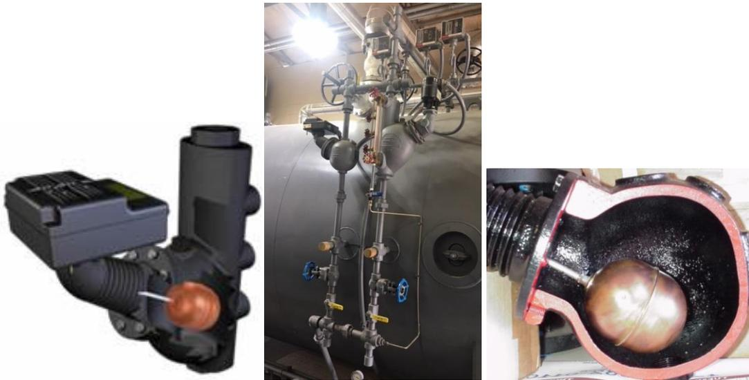
**You must blowdown the water columns daily to flush the sludge and sediment from the bowl to prevent build-up of mud.**
