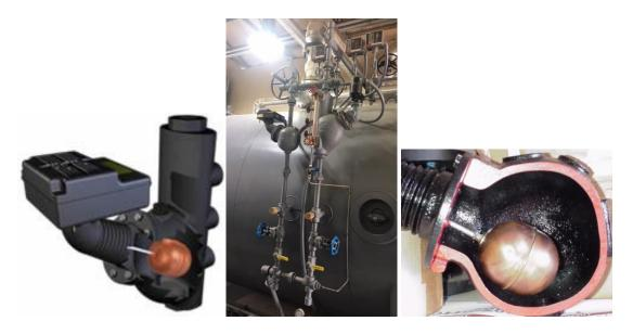
You must blowdown the water columns daily to flush the sludge and sediment from the bowl to prevent build-up of mud.
