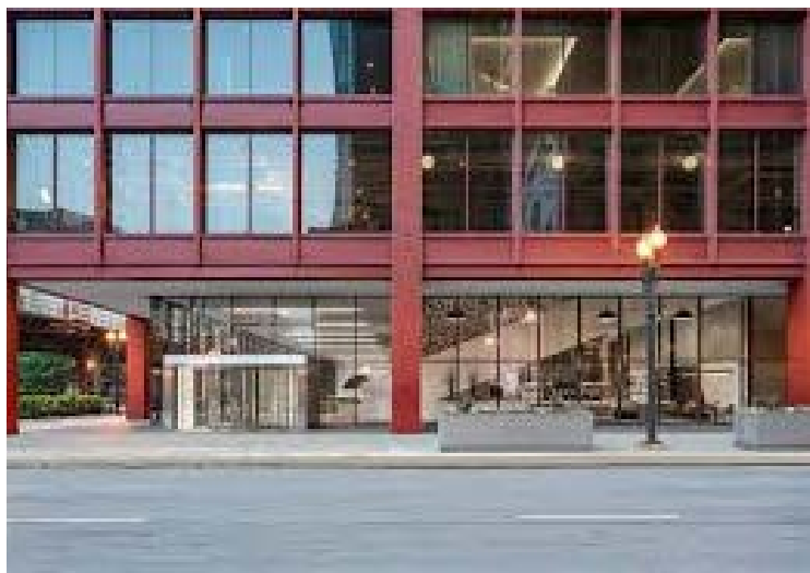
Fig. 35 Ground Floor Exterior View
