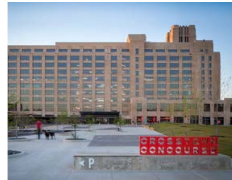
Fig. 9 Overall Exterior View
