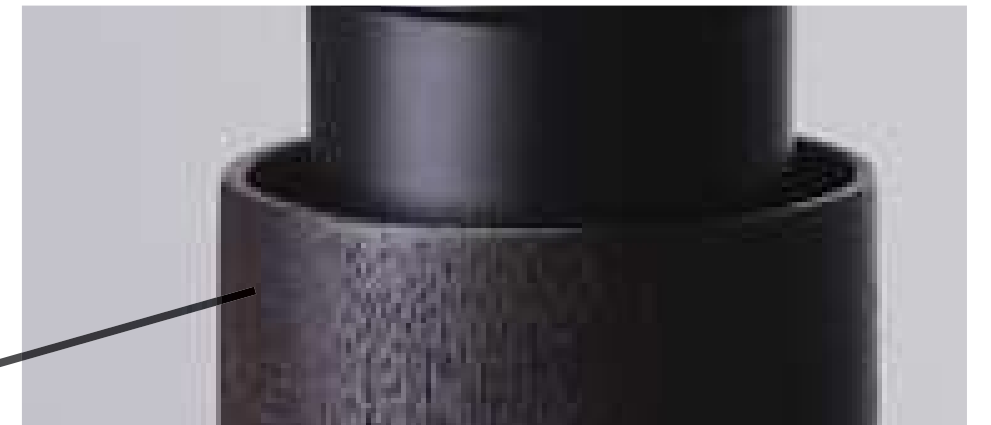
BLACK POWDER-COATED STEEL Metal frame for entry gateway made of steel, then powder-coated and painted black
