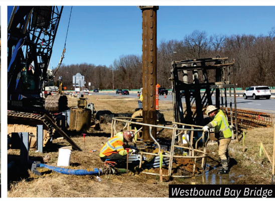
Westbound Bay Bridge
